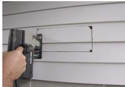
CUT OPENING ALONG MARKED LINES.
